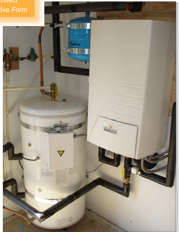
The Daikin Altherma system consists of 2 main components (outdoor unit and hydrobox) that can also be combined with optional accessories such as a water tank and solar thermal kit to ensure ideal water temperature.
