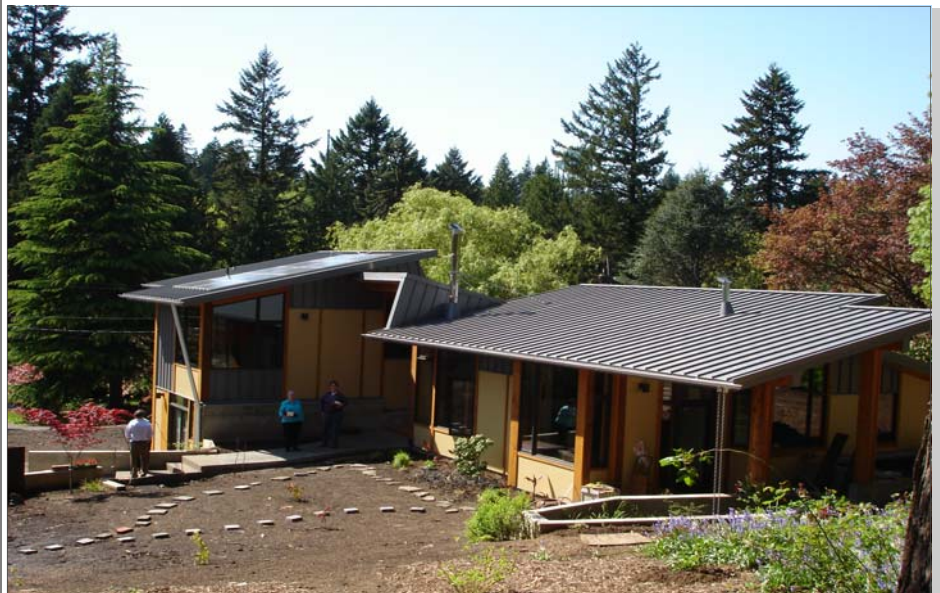
The Bauman-Broussard home, which received a LEED Platinum rating, is the site of the first installation of Daikin Altherma.
